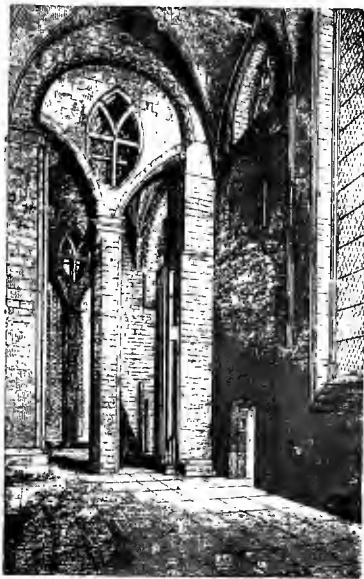
NORTH ARCH OF CENTRAL TOWER, SHOWING MASONRY ERECTED ABOUT 1320.
